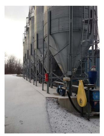
This is a row of silos used to store recycled materials in Bloomfield NY. The conveyer system is used to bring the materials into the plant where is it densified so it can be reused to make more foam. PS foam from our factory is about 30% recycled content.
